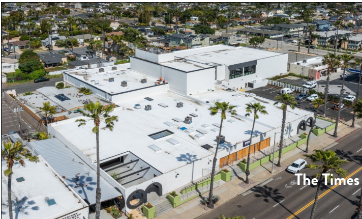
The Taco Stand, Mason Aleworks, and Rumble Boxing Gym are coming to The Times building at 1722 S Coast Hwy.
